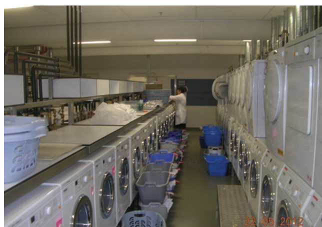
Laundry lab Q-building
